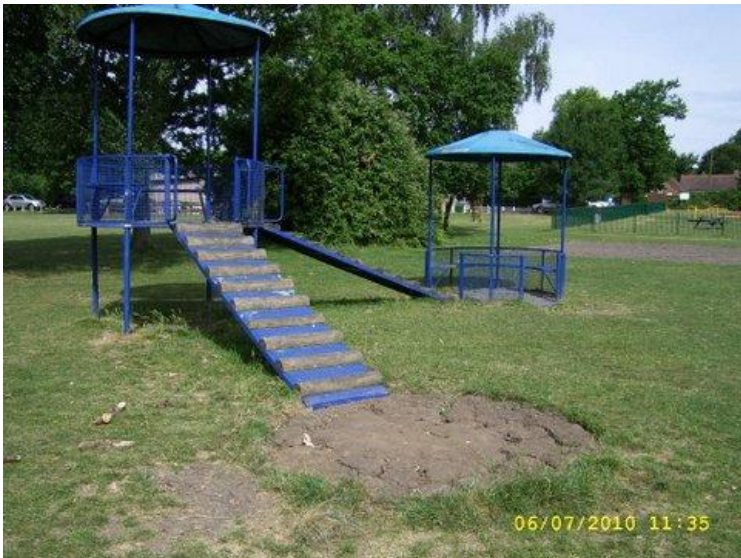
Current arrangement with one module missing which was uprooted in 2010 and rolled away to the woods on the far side of the football fields. The higher unit has been fire damaged and had to be repaired following the front handrail assembly being wrenched off. The unit removed weighs 250kg and is about 1.8m wide x 2.5m tall.
